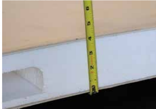
4" thick roof With built-in insulated A/C ducts.
