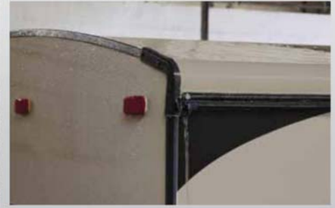
TPO Roll Over Roof
